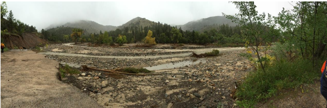
Panoramic from where a fire station once stood. Photo courtesy Jim Houck, CO-TF 1
